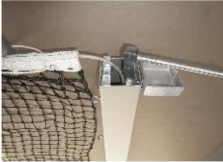
Then pull the hook down with the help of the wrench until the lateral net meshes are close to the upright.
