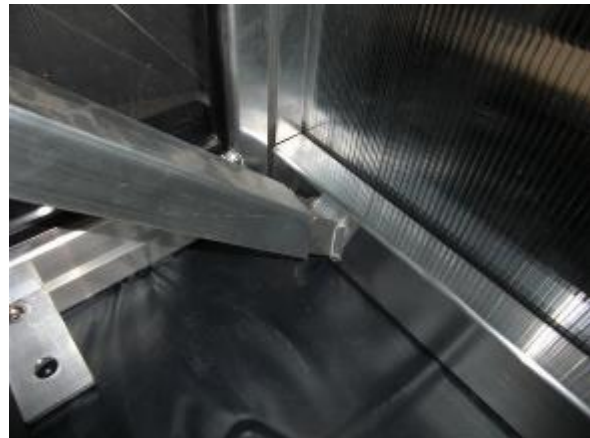
Picture 30: Stick middle supports on the spigots welded at the rear wall. Both middle supports with 5 nuts have to be inserted on the exterior spigots. Position each rear nut M8x20 over the 9mm hole and screw machine screw M8x45 from below.
