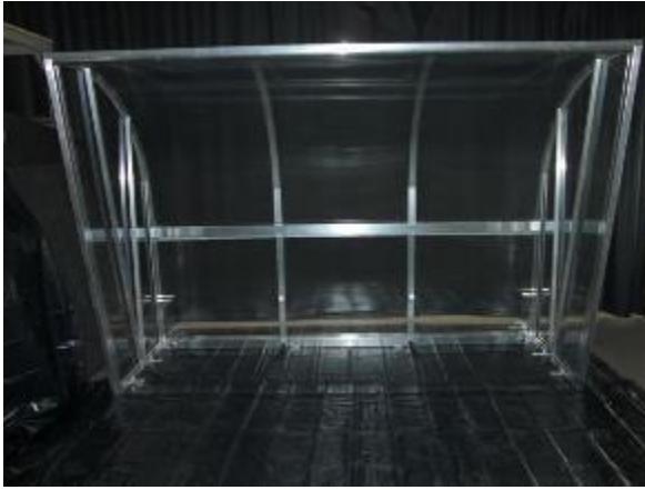
Picture 27: Erect cabin again.
