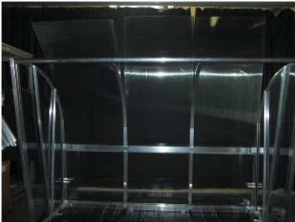
Picture 21: Remove protection foil of remaining hollow chamber plates. Stick them in the angles mounted before: At the outside one plate each 970 x 1,990 mm and in the middle plates of 990 x 1,990mm (1 for 3m cabin, 2 for 4m cabin and 3 for 5m cabin).
