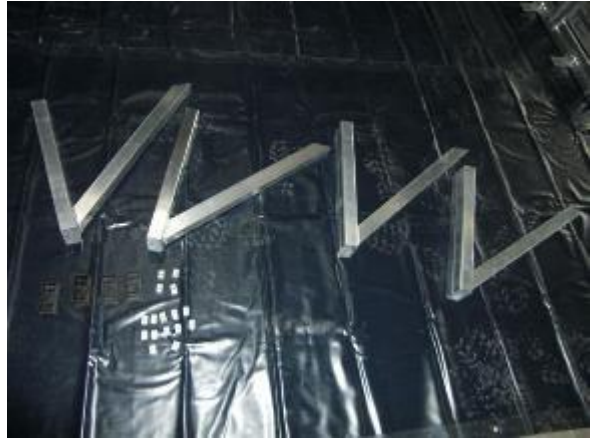
Picture 28: Prepare installation of bench: Middle supports, caps and nuts.
