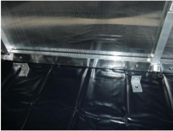
Picture 7: Erect rear wall. Choose two of the prepared rounded head screws to fix ground anchors.
