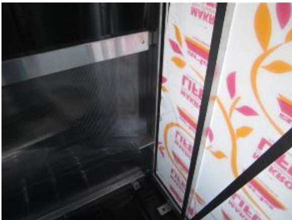
Picture 11: Erect side parts and rear wall and insert plates.
