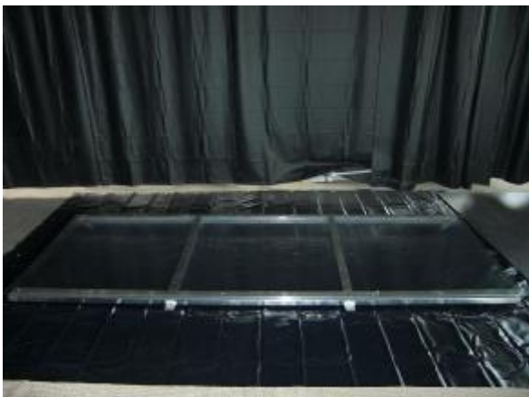
Picture 5: Lay flat aluminium bars 50x2mm on rear wall (for 2m cabin: 2 x 2900mm/ 2 x 880mm; for 4m cabin: 4 x 1950mm/ 3 x 880mm; for 5m cabin: 4 x 2450mm/ 4 x 880mm). Adjust them so that the holes are congruent with the pierced holes of the hollow champer plates.
