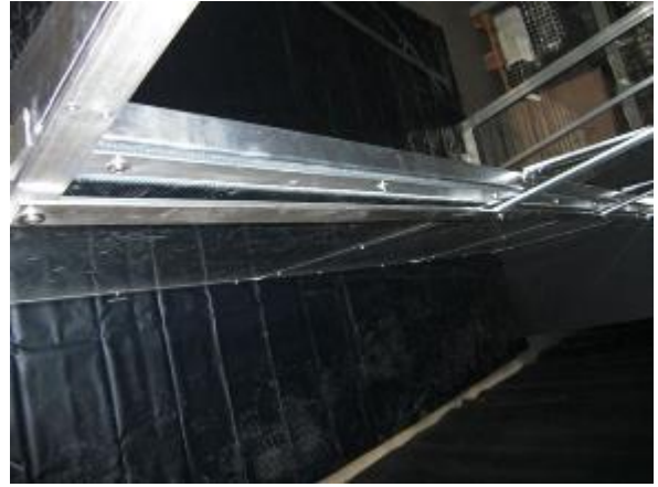
Picture 20: Fix angles 40x30x4mm at both side parts and at roof arches (at the back). Use rounded head screws DIN 7380 M8x16 and washers DIN 9021 Ø 8.4 mm. Attention: only fix screws slightly
