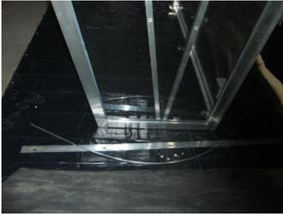
Picture 19: Unscrew roof arch of flat bar 50x2mm mounted at the side part. Also remove flat bar 10x5mm. Put aside both parts as well as screws and washers. The existent spacer blocks were only used for transportation purposes and are no longer necessary.
