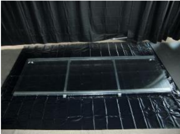
Picture 3: Lay down rear wall, remove protection foil of hollow chamber plates 990 x 970mm and apply plates (3 for 3m cabin, 4 for 4m cabin and 5 for 5m cabin)
