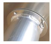
To fix the plug plate stick threaded eye from the reel tube side through the <u>flat</u> hole of reel tube flange and side part (see left picture) and screw it <u>slightly</u> into the plate.
