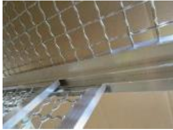
Guiding rail of door in the top part
